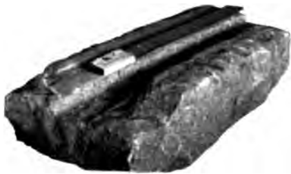
Section of old stone rail used on Kentucky Midland Railroad, from photograph of the original in possession of the Kentucky Historical Society at Frankfort.
